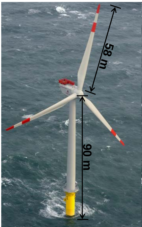
5MW Wind turbine
