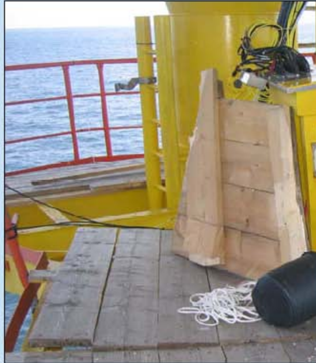
Fig. 1: On 9 November 2007, broken wooden planks on the working platform 15 m above chart datum (left). Basement of the FINO 1 research platform and location of the working platform.
