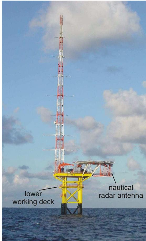
Figure 2: The FINO 1 platform. The nautical radar antenna used for the WaMoS II measurements is installed below the helicopter deck .
