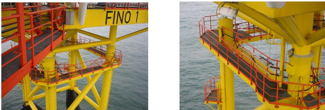
Figure 9: Pictures of the FINO 1 platform showing the damages due to wave impact. (©BSH)
